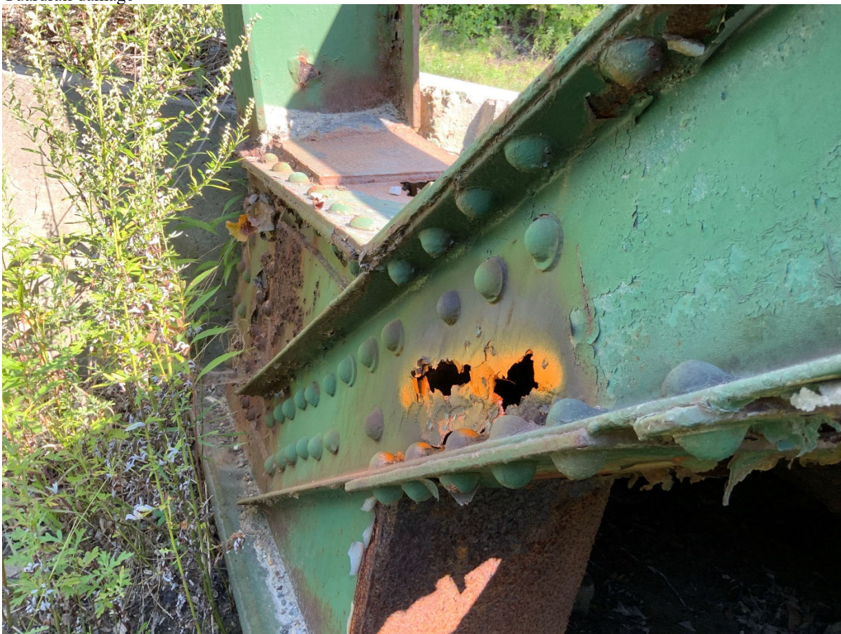
Girder Section Loss
