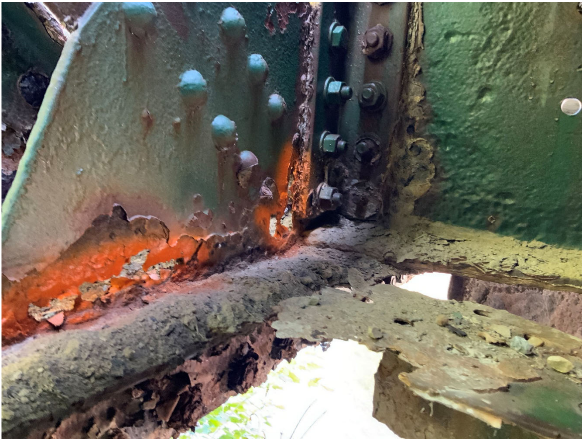
Gusset Plate et al. Section Loss / Separation
