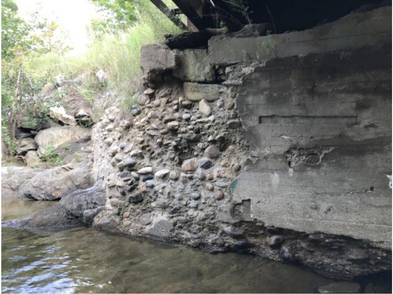
Figure A5: View of Abutment 1 and bedrock exposed running under abutment.
