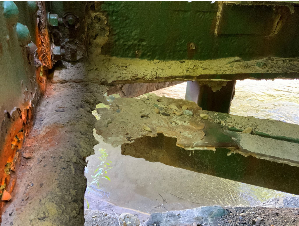
Section Loss / Separation
