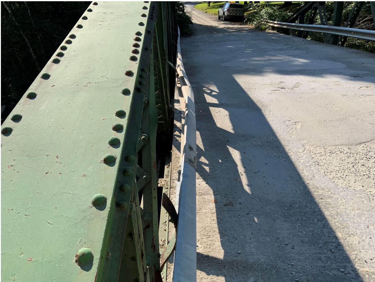
Guardrail damage
