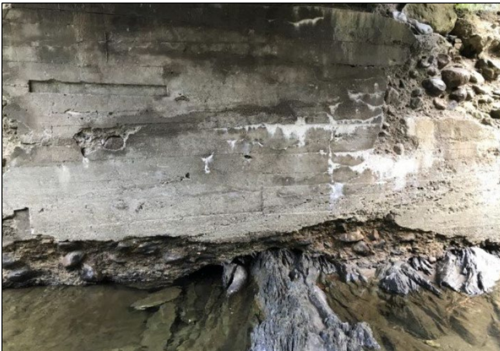
Figure A4: Bedrock exposed under Abutment 2.
