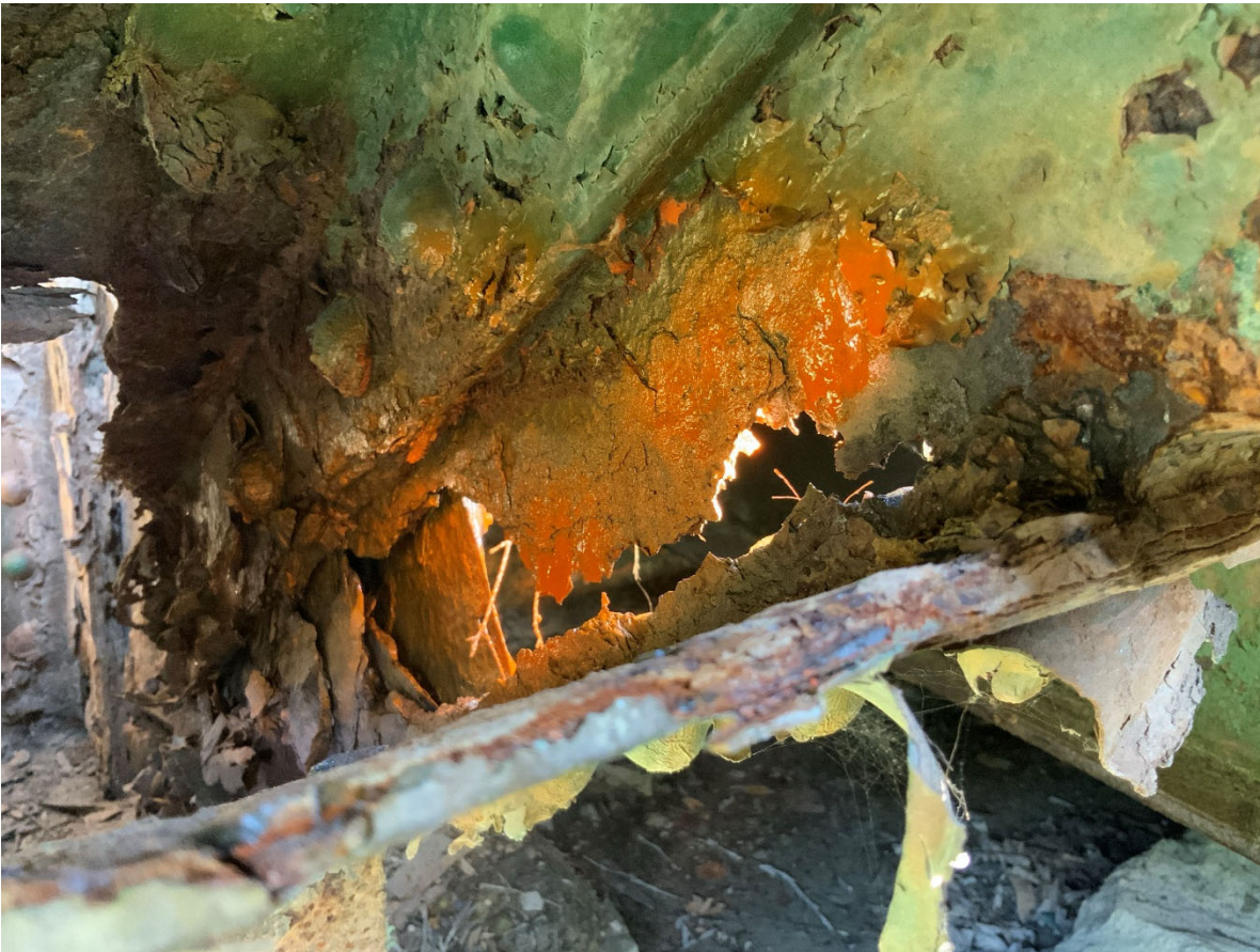
Girder Section Loss
